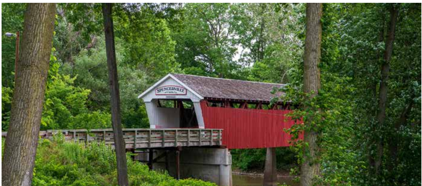
The historic Spencerville Covered Bridge in DeKalb County, Indiana, was built in 1873 and spans the St. Joseph River. In 2021, it was identified as a top priority among the thousands of rural bridges in the United States worthy of repair in President Joe Biden's "American Jobs Plan."
